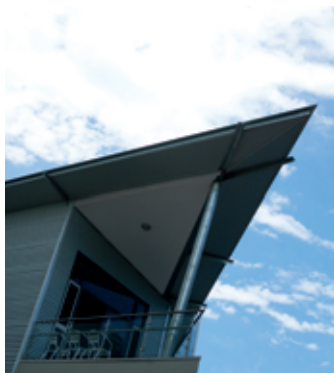
The Deck Bridge
